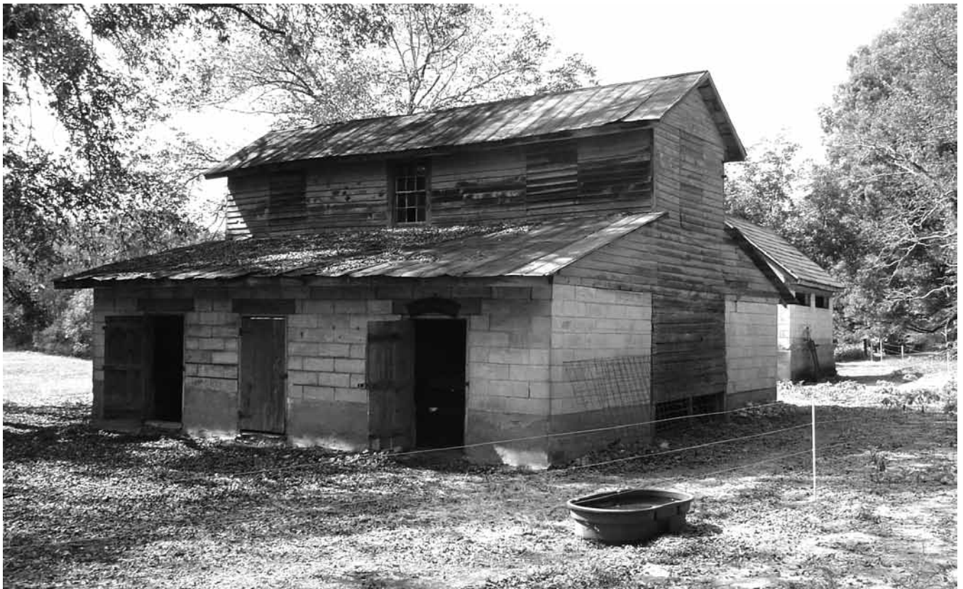
Photos taken on the Shields-Ethridge Heritage Farm. Owner, Ira Ethridge was the brother of Scott Ethridge. Top photo: Cotton gin built circa 1910 using Miracle Ho'Low Blocks. Bottom photo: Mule barn, circa 1916 of blocks by Scott Ethridge
