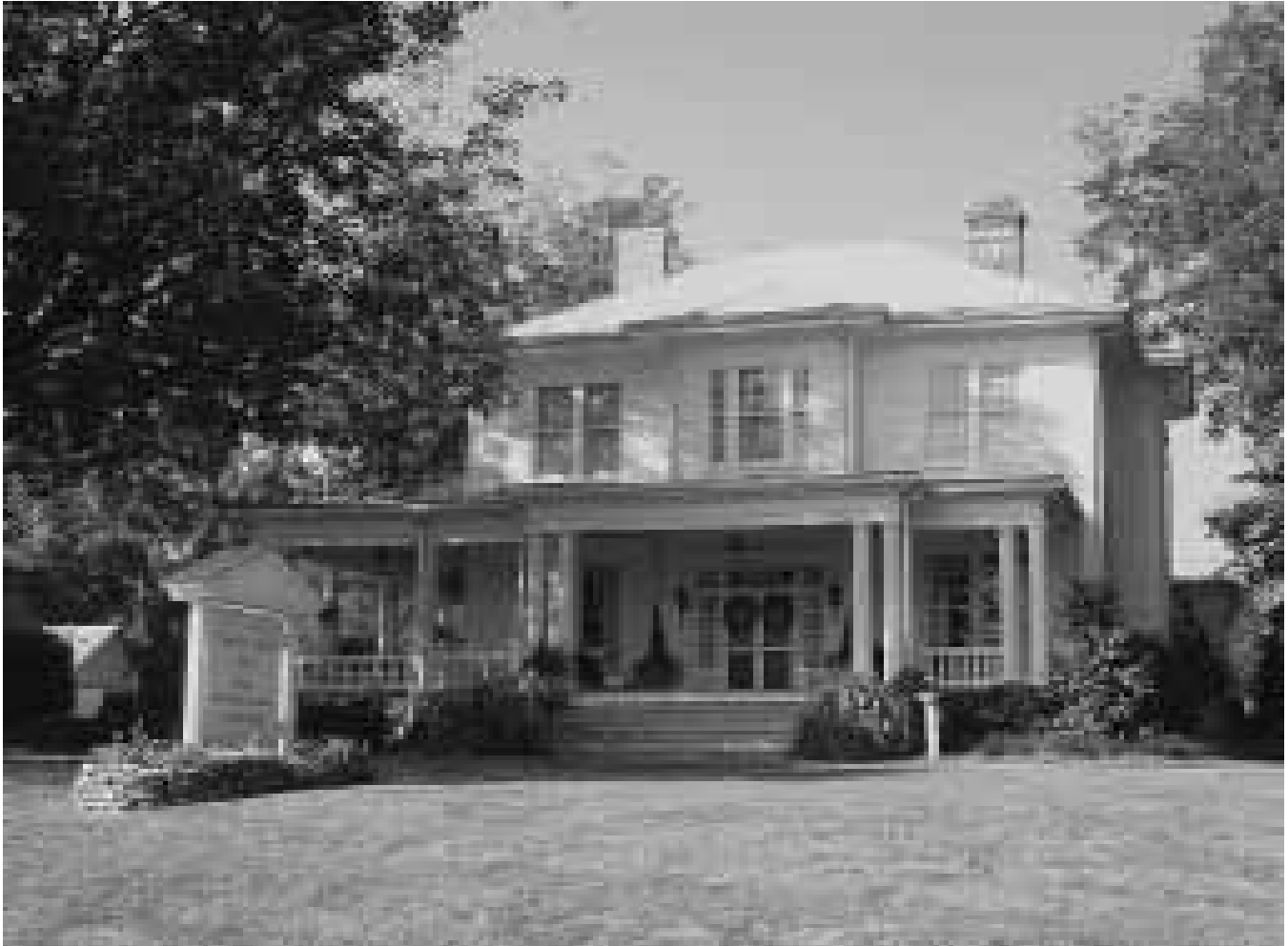
Braselton -Stover House built by Green Braselton, 1918
