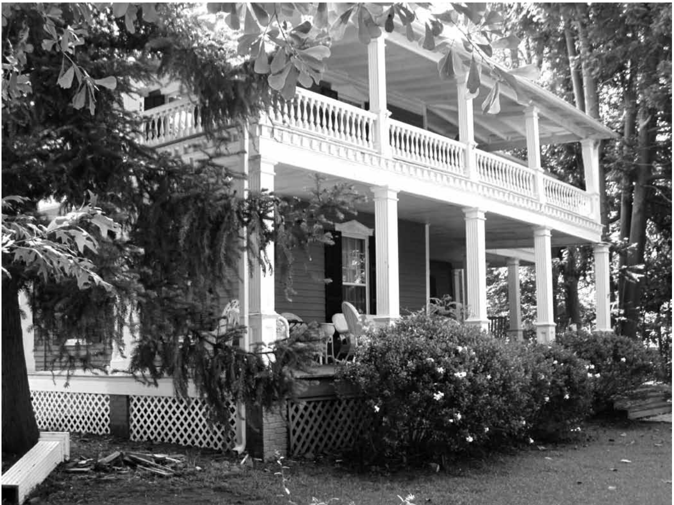
Niblack-Evans House - Storey Street, Jefferson . A plantation home that fronted several thousand acres
