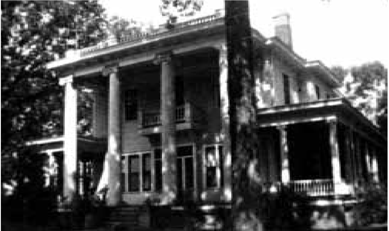
The Braselton City Hall was the former home of the first mayor of Braselton, William Henry Braselton. Built in 1909, it was renovated this year for a city hall and community center.
