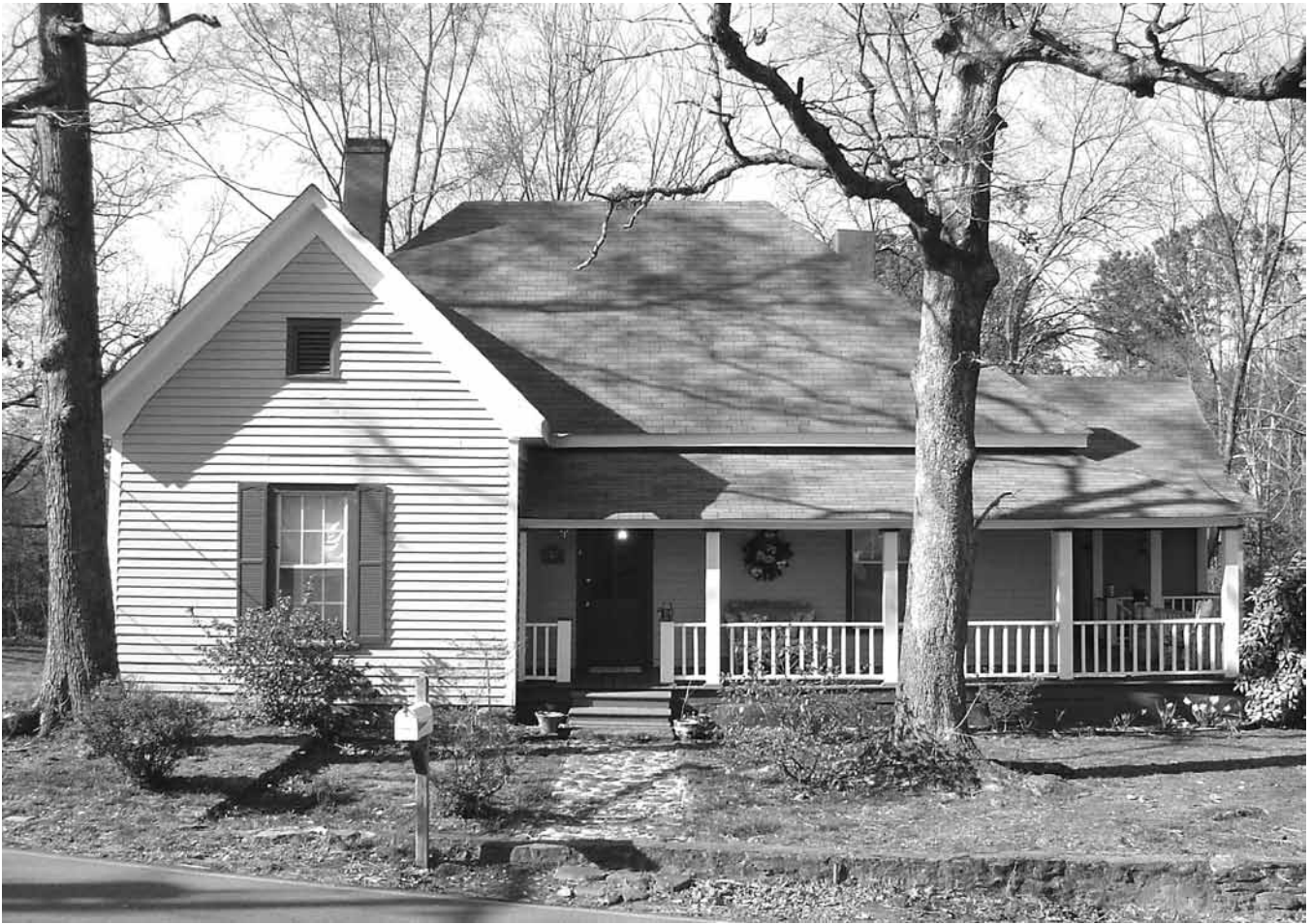
Photograph of the Hardy-Purcell house built circa 1905
