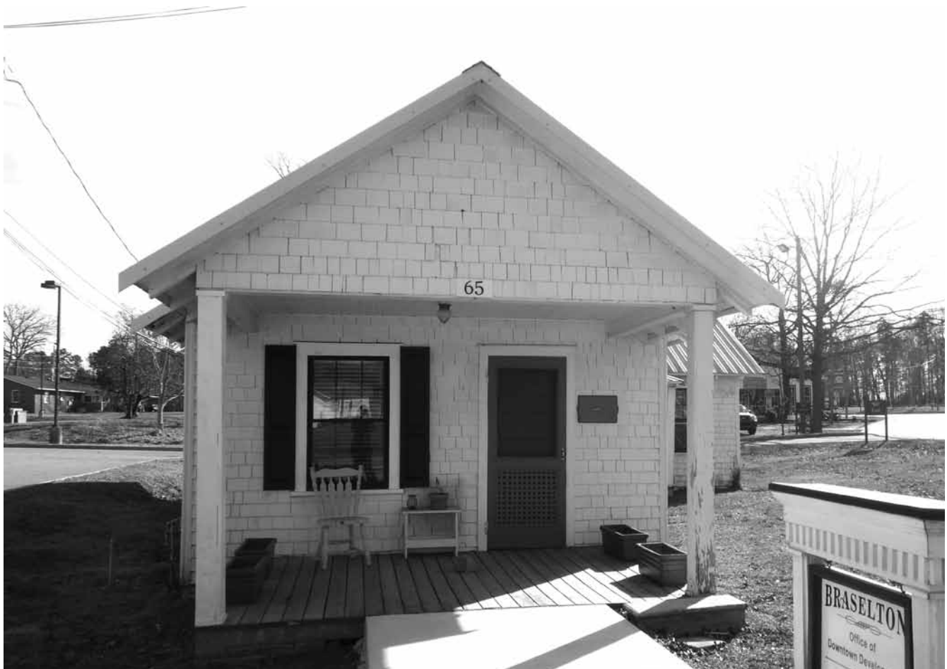
Braselton Downtown Development Office was built as the Home Economics building for Braselton Highschool in the early 1920's
